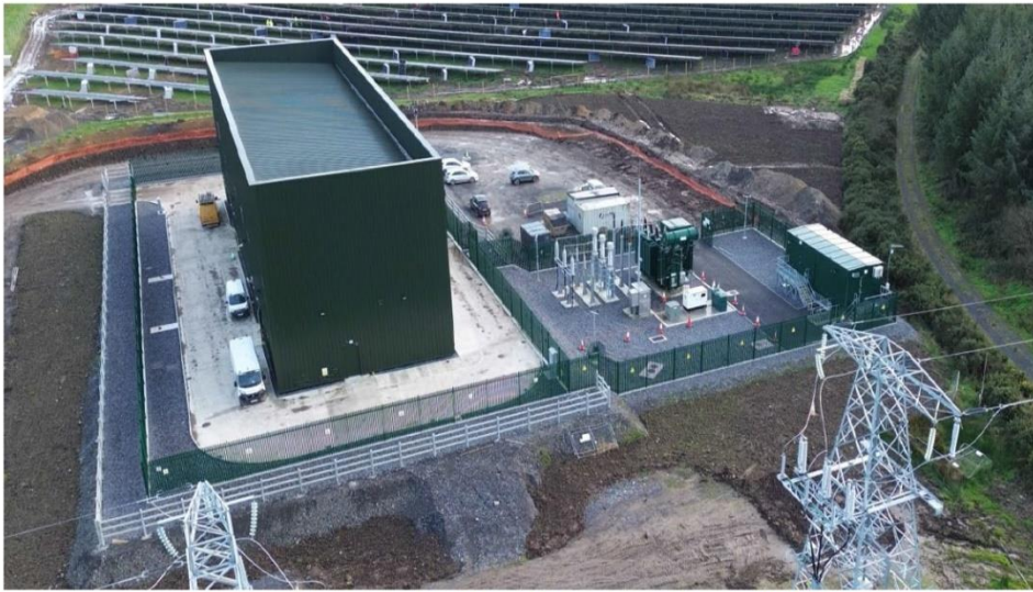
Figure 2-1: Typical 110kV GIS Station Layout (Source: H&MV)
